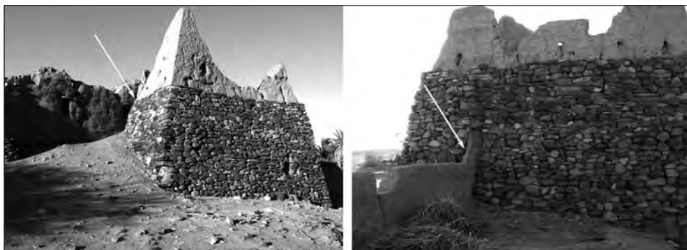
Fig. 13. Kissenfarki East: fortifications of a post-medieval fort; arrows indicate construction phases (Photos M. Drzewiecki)
