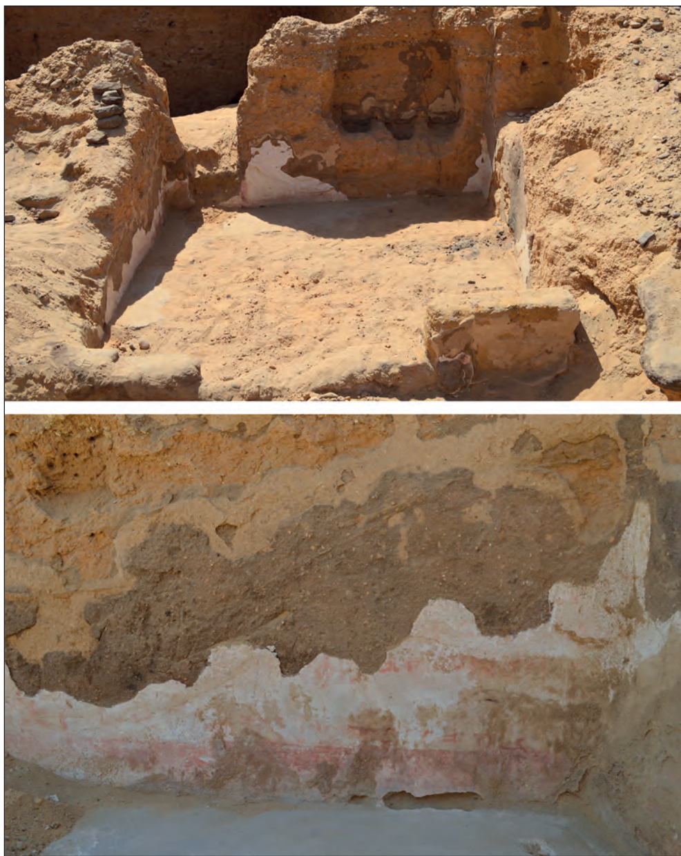
Fig. 8. EE.50.3.2: top, view of the room toward the entrance in the south wall, note patch of lime plaster preserved just above the floor next to the entrance and niche with three circular hollows in its floor; bottom, remains of lime plaster with a painted inscription on the east wall (PCMA Naqlun Project/photos W. Godlewski)
