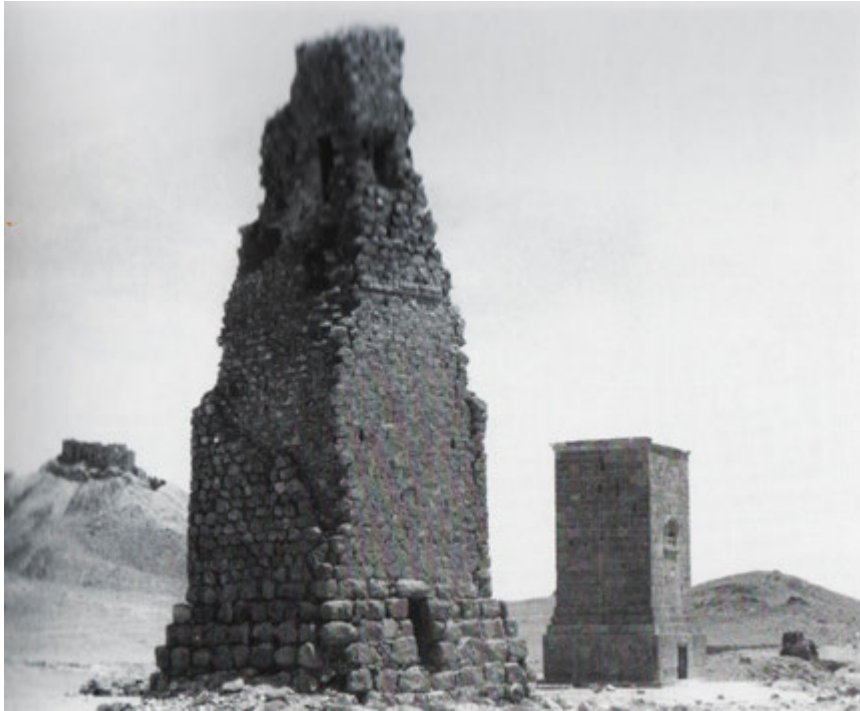
3. The tower of 'Atenatan (7 BC) and, behind, the tower of Elahbel (AD 103)
